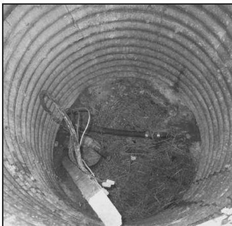
Drilled well in a pit.
